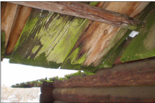
Fig. 7. Effect of excessive moisture – barn from the village Bukowa.
