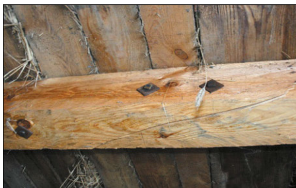
Fig. 1. Strengthening the joist – wood farmhouse from the village of Niemce.
